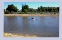
The Nacimiento recharge basin allows water to percolate into the groundwater basin, replenishing water storage.
